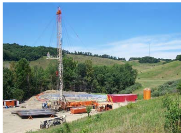
Drilling operations at the Ohio CO 2 sequestration test well in Tuscarawas County, Ohio. Both CO 2 storage units and natural gas were discovered in this well.
